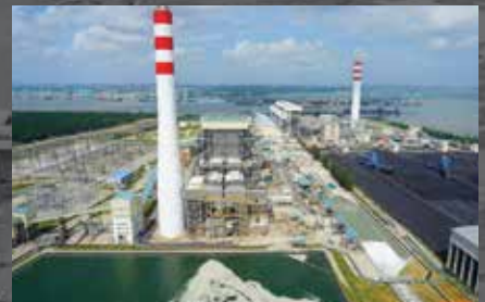
TANJUNG BIN POWER PLANT Electrical and instrumentation work for 3x700MW (2006) and 1000MW (2016) Coal Fired Power Plant
