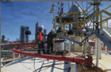
GAS PROCESSING PLANT 4 (GPP4), TERENGGANU Tank Internal & External Refurbishment Works
