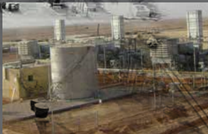
AL-JAL AMID (SAUDI ARABIA) Mechanical, Electrical & Instrumentation works For 3x25MW Gas turbine Power Station & Substation
