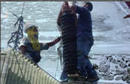
CHENDEROH HYDRO POWER PLANT Refurbishment of 11.5MVA Generator step up Transformer
