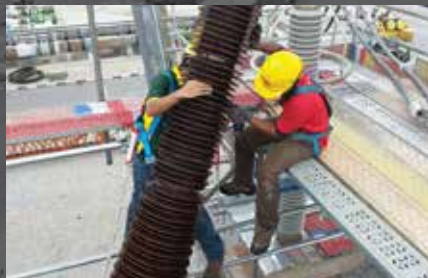
MANJUNG POWER PLANT Major Service of 1050 MVA Generator Transformer
