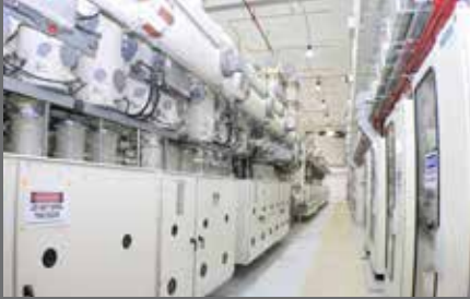
PETRONAS P14-1001 RAPID, PENGERANG Construction and Commissioning (CC) of 275kV GIS Electrical Equipment Installation
