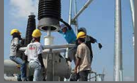
PMU SUBANG TOWN CENTRE 275/132/33KV GIS Installation and Testing works of 275/132/33kV GIS at PMU Subang Town Centre
