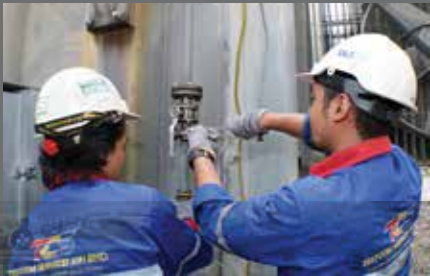
PMU SERDANG 132/33/11KV Transformer oil regeneration and reinhibition services carried out online at PMU Serdang
