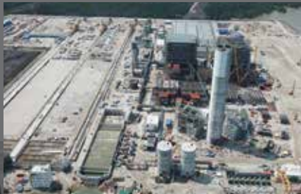
JIMAH POWER PLANT Electrical & Instrumentation works for 2x700MW (2007) and 2x1000MW (2018) Coal Fired Power Plant
