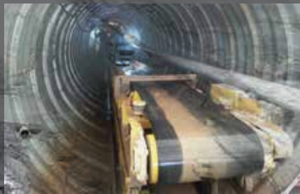
KRUENG ISEP, ACHEH, INSONESIA Engineering, Procurement and Construction works for 20MW Run of River Hydro Power Plant
