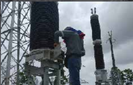
PMU PERMAS JAYA 275/132kV Testing & Commissioning of 2x275kV Overhead Line Feeder
