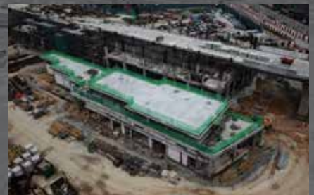
MRT LALUAN 2: SUNGAI BULOH SERDANG-PUTRAJAYA (SSP) S201: Construction of elevated stations and substations and other associated works at Damansara Damai, Sri Damansara West, TPSS4, TPSS5, substations, Damansara Damai utilities building and Sri Damansara East Main Station
