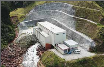
TEMBAT HYDRO POWER PLANT Electrical & Mechanical works for 2 x 7.5MW Tembat Hydro
