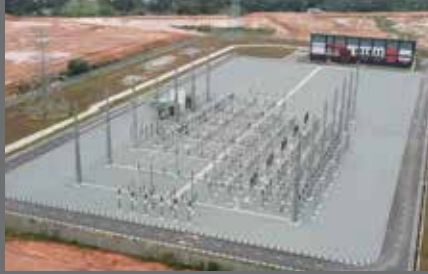
PMU SENAI HI-TECH 132/33kV AIS Supply/ install & commission for 132/33kV Substation and associate civil work
