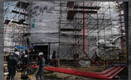
GAS PROCESSING PLANT 2 (GPP2), TERENGGANU Tank Refurbishment works for Petronas plant Rejuvenation and Revamp 2
