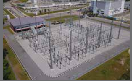
PMU SETIA ALAM 132/33kV AIS Supply/ install & commission for 132/33kV Substation and associate civil work
