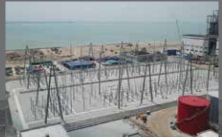
JIMAH EAST 500kV AIS Erection and testing works for 500kV Jimah East AIS Switchyard
