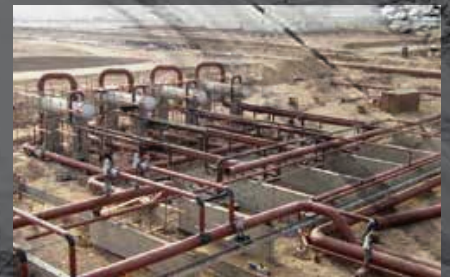
BASHAYER-2, SUDAN Electrical & Instrumentation works For Bashayer-2 Oil Export Marine Terminal
