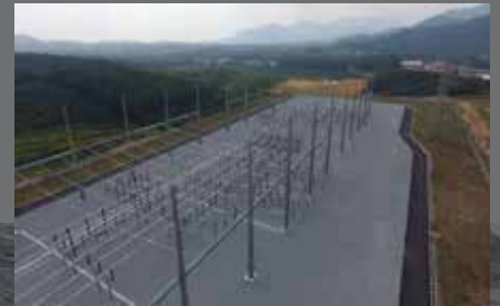
PMU TAPAH 275KV Establishment of 275kV Tapah Substation, including associate civil work
