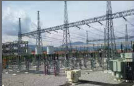
PMU PAPAN 275/132KV Rehabilitation works for 275/132kV Papan including associate civil work
