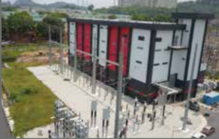
PMU KL (NORTH) 275/132/33kV GIS Supply/ install & commission for 275/132/33kV GIS Substation and associate civil work
