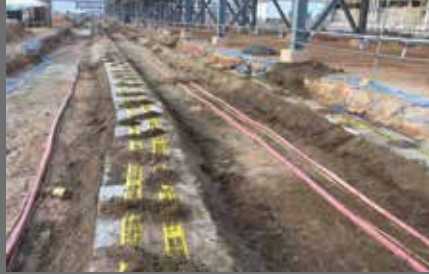
PETRONAS P14-1200 RAPID, PENGERANG Construction and Commissioning (CC) of 33kV and Below Distribution Substation Feeder, Cable Laying, Jointing and Termination at Gas Insulated Substation (GIS)
