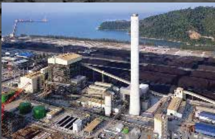
MANJUNG POWER PLANT Cable-Laying & Termination for 1x1000MW (2014) and Electrical & Instrumentation works for 3x700MW (2003) Coal Fired Power Plant
